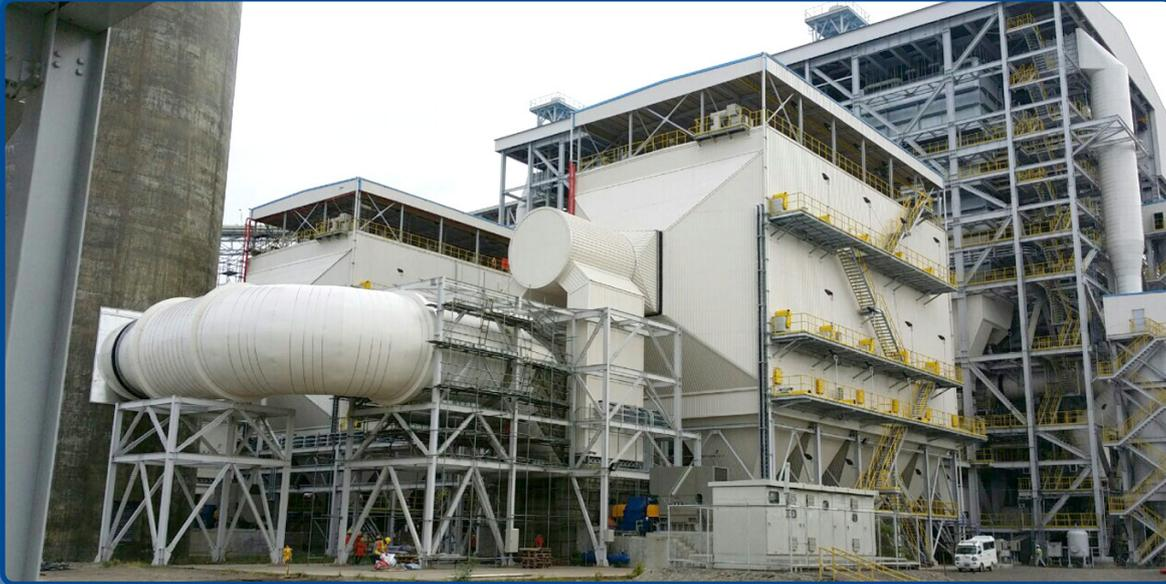
With an Electrostatic Precipitator (ESP), direct high voltage is applied to create a corona discharge to charge particles suspended in the gas and collect them through electrostatic attraction. An ESP is useful in removing particles in the sub-micron range which are difficult to capture with gravitational or centrifugal force.
